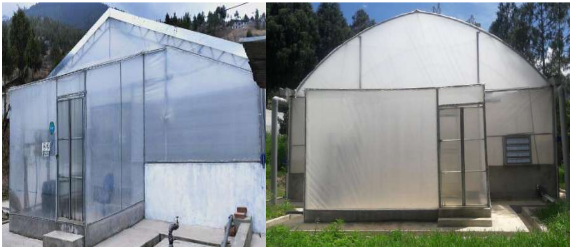
Figure 20. Prefabricated Greenhouse for hydroponics
