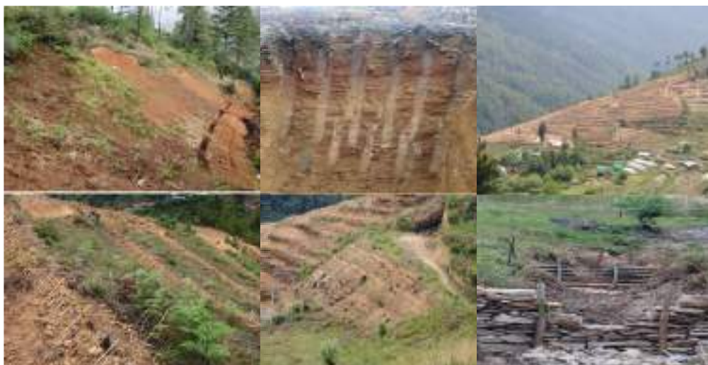
Figure 25 Different SLM technologies established at the technology park
