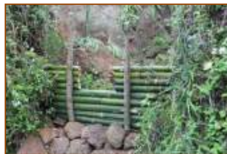
Picture 30: Check dam construction
