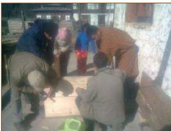
Picture 22: Electric dryer construction in process
