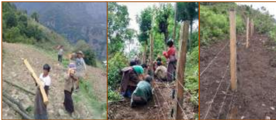
Picture 39: Installation of electric fencing at Pangthang, Wangphu Geog. Samdrupjongkhar
