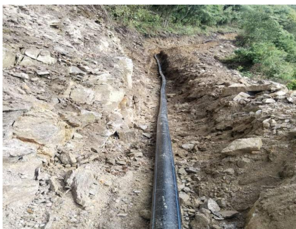
Trench laying of HDPE, Gayrikha scheme in Haa
