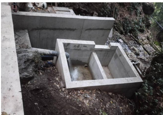
Side intake at Khangma Scheme in PemaGatshel
